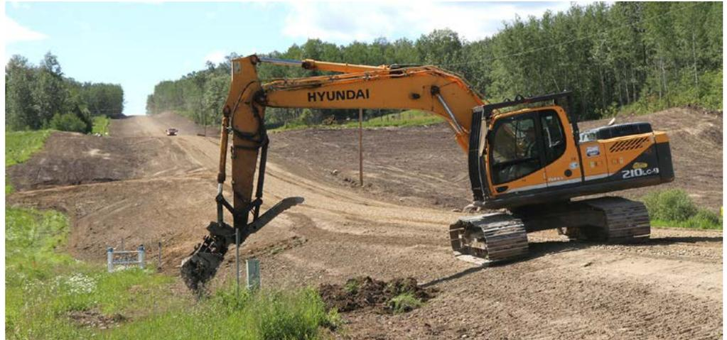
**ROAD UPGRADES** - a track hoe operator puts finishing touches on Township Road 650 near Meanook. The road was upgraded to reduce its grade and improve drainage.
