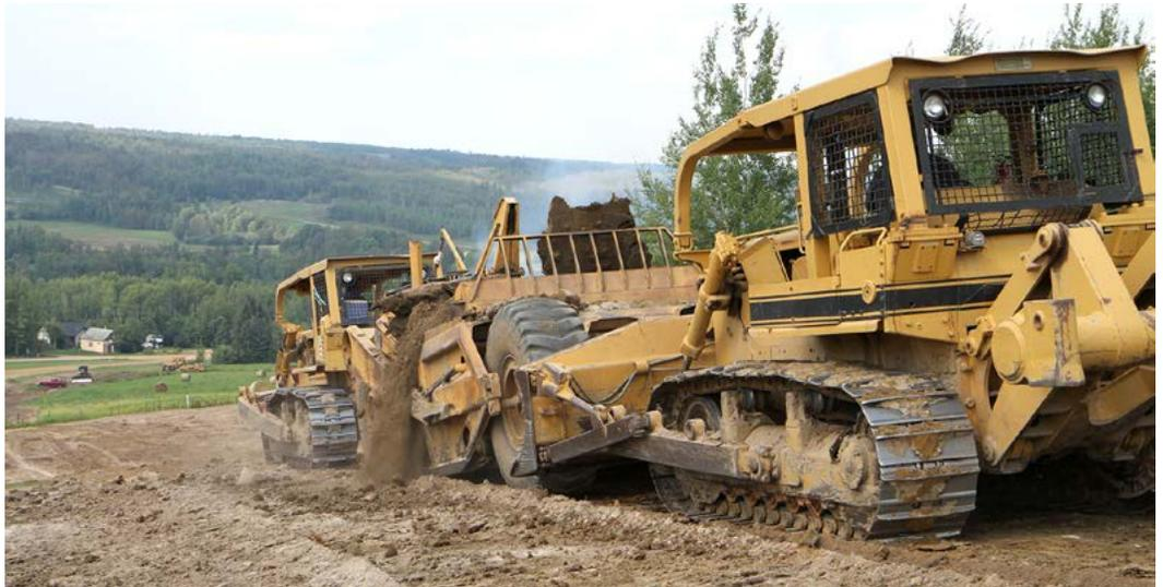
Heavy equipment works to load roadbase material at a road construction site in Meanook. The road was due for an upgrade and was experiencing drainage issues making the road difficult to drive on during periods of lengthy rain.
